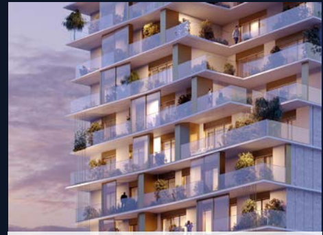
Milan Feel UpTown - Via Pier Paolo Pasolini, 3, 20151 Milano 600 apartments, all 6 Comelit product families installed
