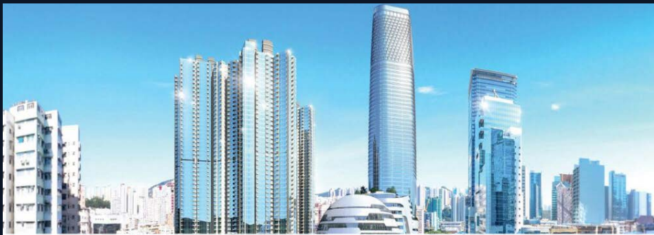
Hong Kong Grand Central - 33 Hip Wo St, Kwun Tong, Hong Kong 4 towers, 1999 apartments, 30 external units
