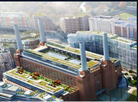
London Battersea - Circus Rd W, Nine Elms, London SW8 5BN 865 apartments, 50 external units, 7 logifire panels networked with over 100 network zones per panel
