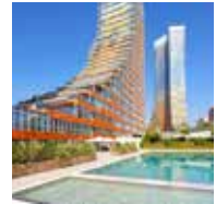
Turkey, Istanbul Varyap Meridian Color Planux monitors. Integration with Fire Alarm System and panic messages. Integration with additional CCTV cameras - Burglar alarm
